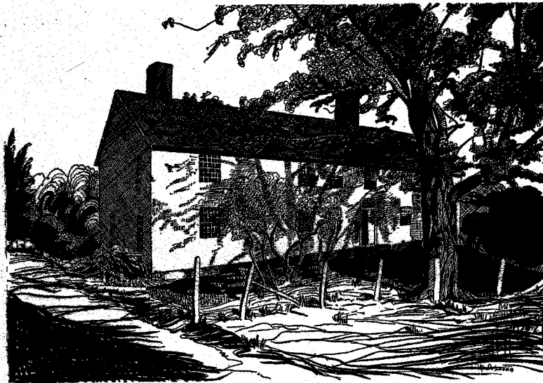
THE ROSE HOUSE ( circa 1720), BUILT NEAR SIBBIE'S HILL BY JONATHAN ROSE, GREAT-GRANDSON OF ROBERT ROSE OF BRANFORD. Rooms from this house have been installed in the Yale Gallery of Fine Arts. The pen and ink drawing was made by the great-great-great-granddaughter of the builder.
